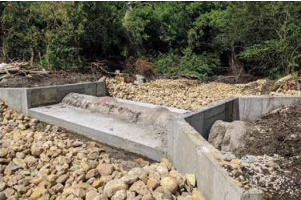
One of the pipe dam locations completed during construction in 2020.
